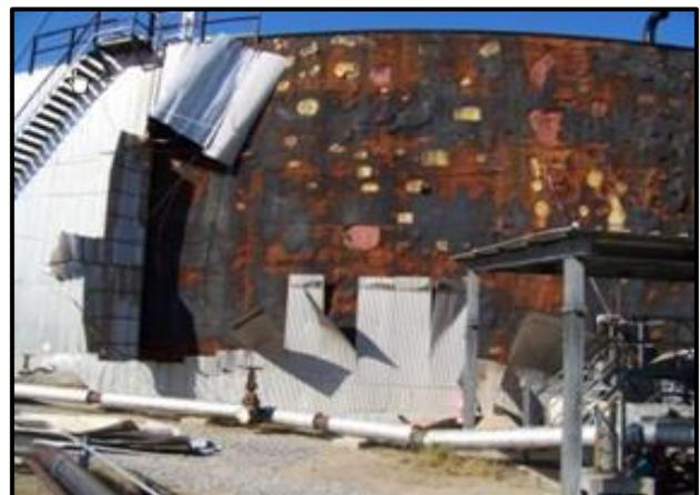
Fig 4 CUI Damage on a Storage Tank
